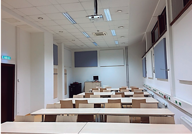
Figure 11. Ten prefabricated panels cladding large parts of three walls of room i14 were meant to improve the acoustical comfort for lectures and communication.
