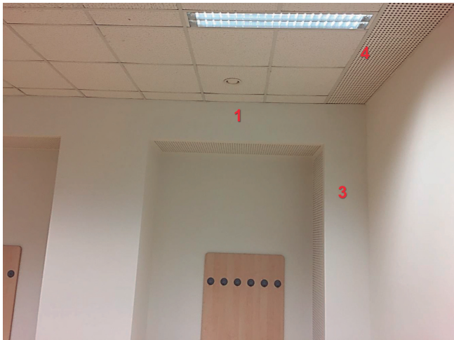
Figure 16. Absorber packages behind perforated gypsum plates within the cavity in front of both partition walls accomplish the alternative broadband installations.
