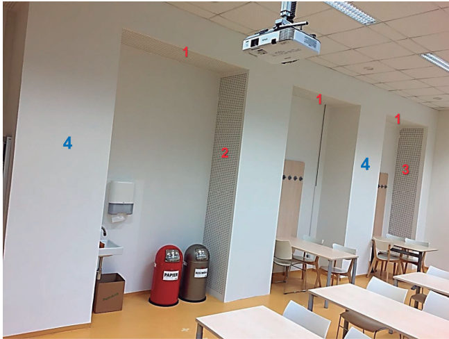
Figure 15. Door-side wall of room i15 equipped with horizontal edge absorbers 1 and vertical coffers 2 (two-sided) and 3 (one-sided) resembling the original protrusions 4.
